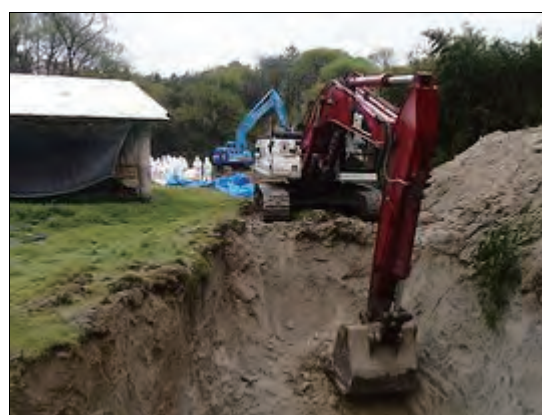
埋却穴の掘削
